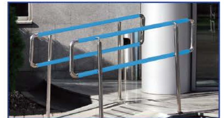
Wheelchair Ramp Railing
